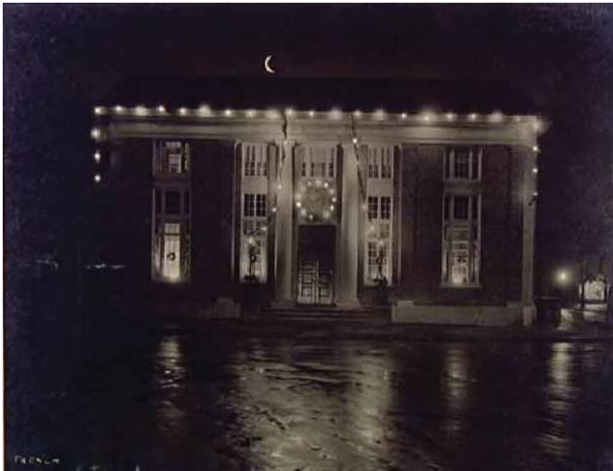
Montclair National Bank, no date. The original window configuration is evident in this photo, which also illustrates the original paneled bronze doors.
